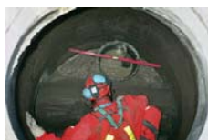
Brønd under reovering.
